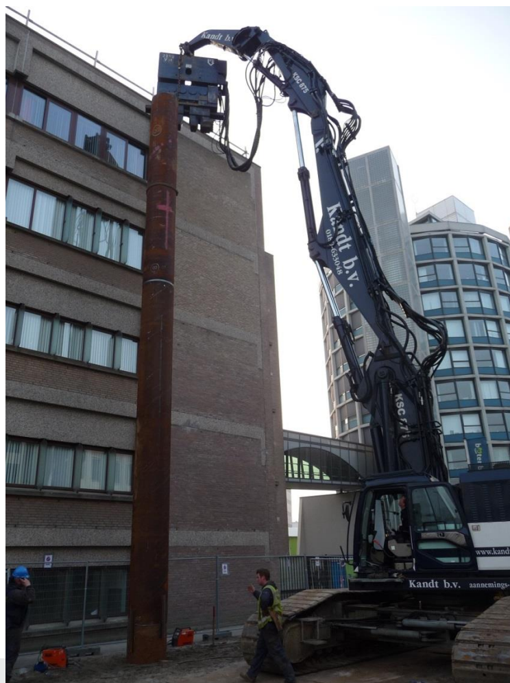
Intrillen stalen casing.
